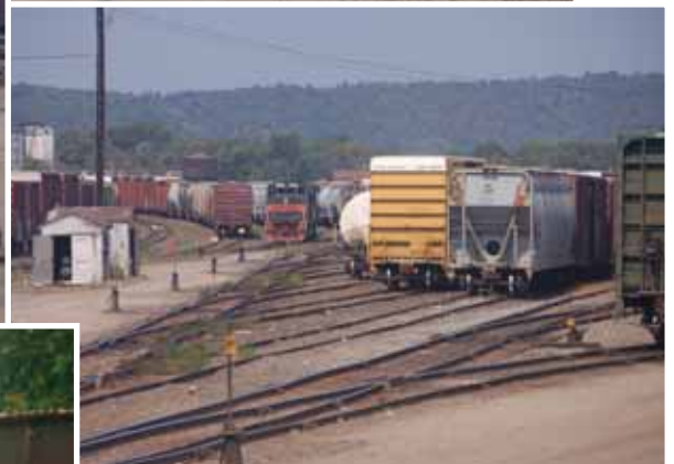
Looking Down the Classification Yard (Westward) Towards the Receiving Yard
