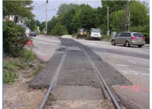
“Before” Facing East
