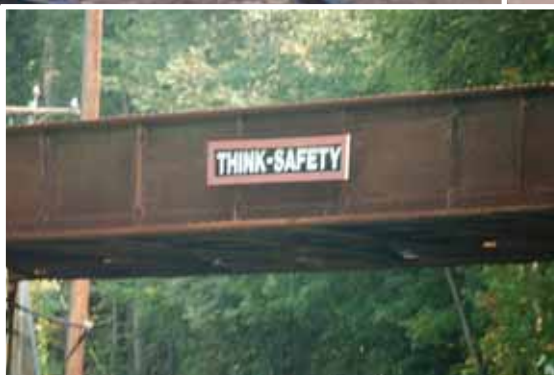
Loop Track Bridge Photo Credits: Ed Motte
