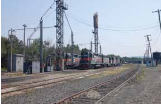
Locomotive Servicing Facility
